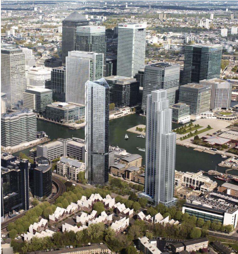
Figure 7. CGI - Meridian Gate (permitted on the left) and 225 Marsh Wall (proposal on the right)
